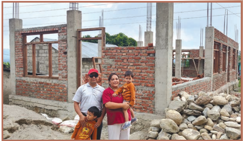
An HCLCN church under construction
