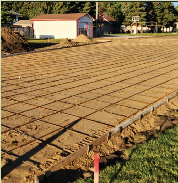
New concrete parking lot going in
