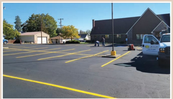
Trinity parking lot resurfacing project.
