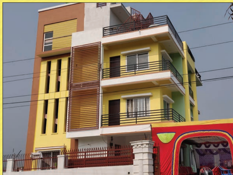
HCLCN headquarters and seminary building.
