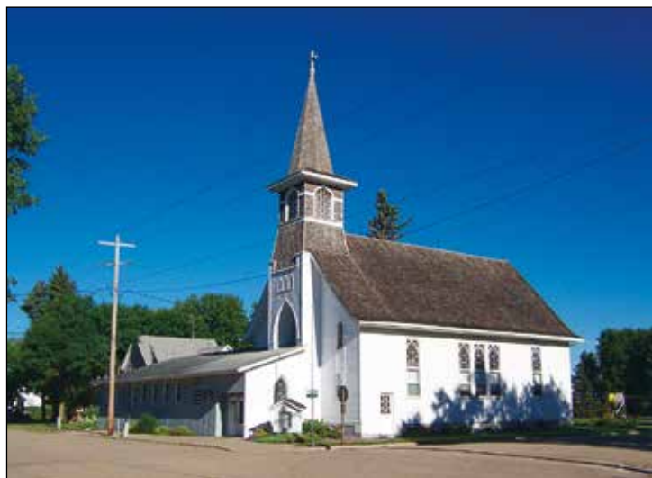
Exterior of St. John's Lutheran Church.
