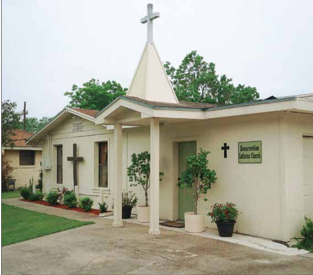
Exterior of Resurrection Lutheran Church.
