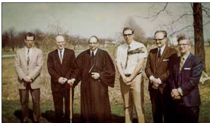
Groundbreaking on April 26, 1970 (Rev. R. E. Schaller holding the shovel)
