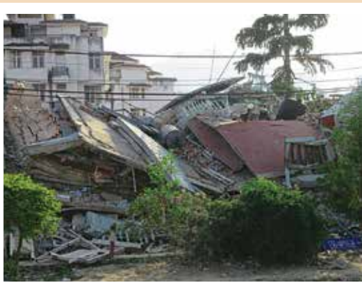
Kathmandu, Nepal. Example of damage caused by the 7.8 magnitude earthquake that occurred on April 25, 2015..
