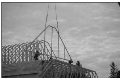
The new AC rafters were raised and the ceilings were finished.
