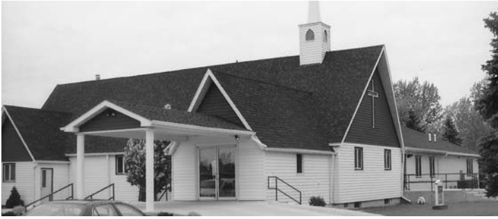
Additions to Trinity Church—a new entry and car ramp to the east, followed by a sizeable fellowship hall off to the west
