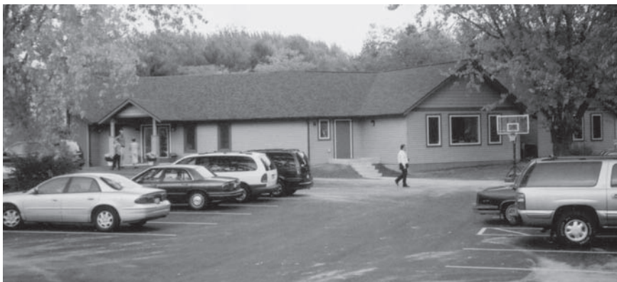
Exterior of the New Addition
