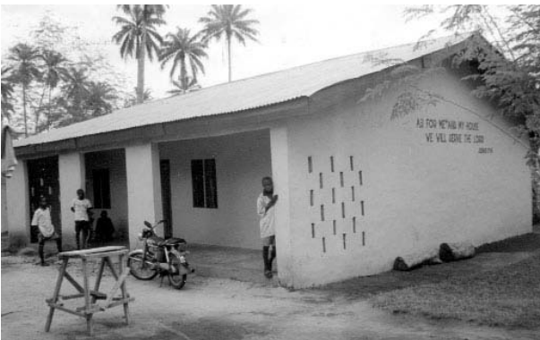
Teacher's House for Pastor Edwin. It is next door to the new house.
