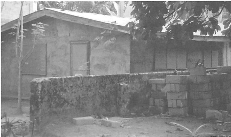
In the Spring, volunteers Larry and Martin Hansen remodeled this house for the second missionary in Nigeria (more pictures, p.19).
