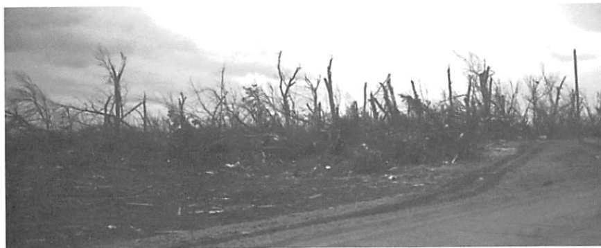
The March 29th tornado in rural Hanska, Minn. took all the buildings on this farm site, leaving only a grove of stumps. No one was injured.
