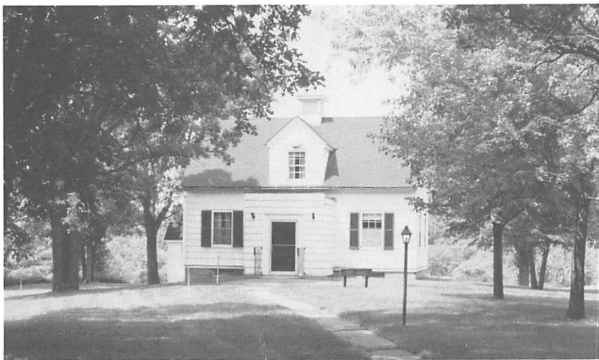
The sun setting on the "Sem House" which is being moved to make room for the new building on our Eau Claire campus.
