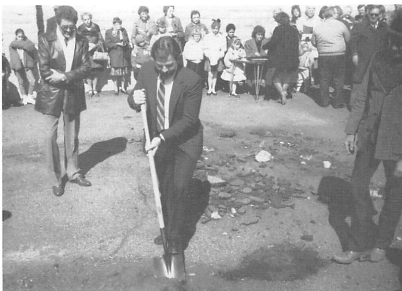
Pastors Dale Redlin and Douglas Libby (with shovel) at ground-breaking of Immanuel's new multi-purpose addition.
