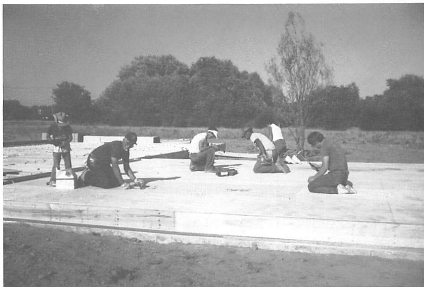
Laying The Foundation
