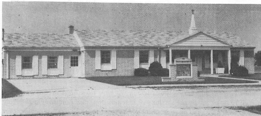
The First Church—Now Remodeled As Parsonage
