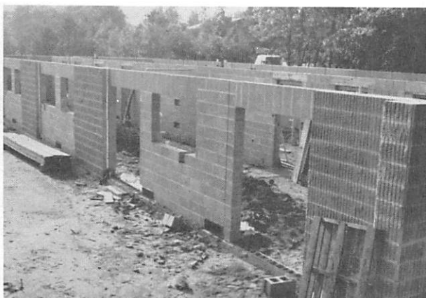
Progress on the Dormitory
