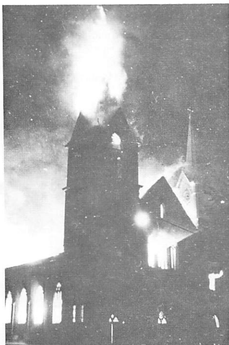
The church during the early morning blaze.
